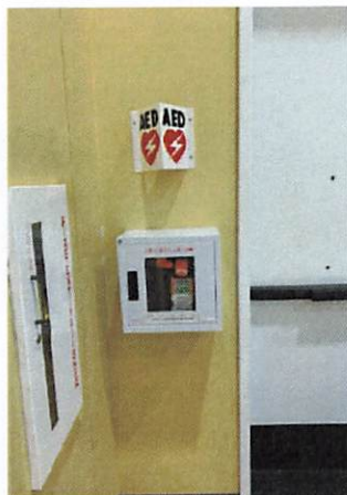
27 Freed 1 st Floor Court
